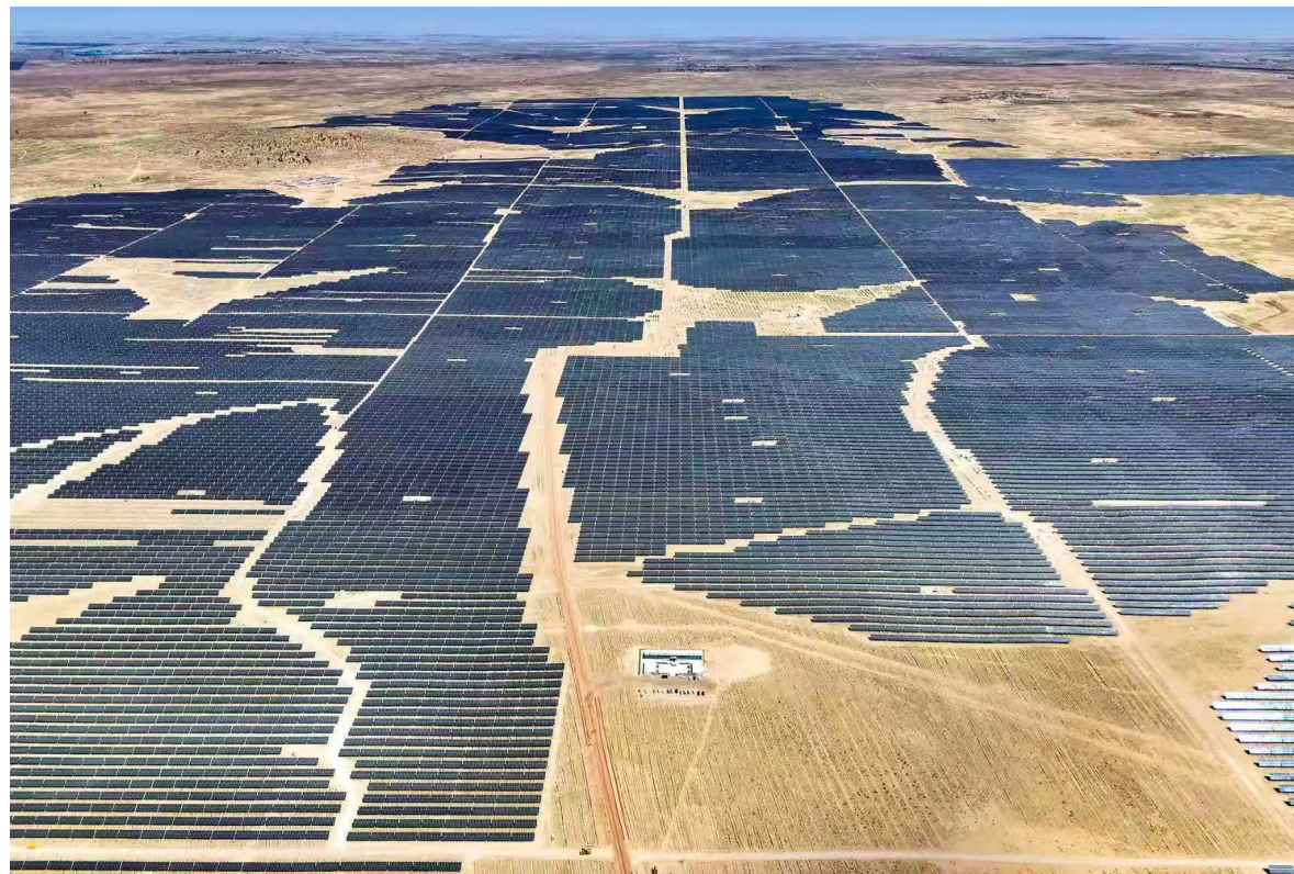
the 1.2 GW Power Plant of Ningxia Yanchi Gaoshawo (Ningguoyun)
